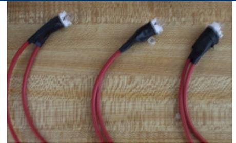
Solder the wires onto the LED contacts, one wire per contact. Afterward, wrap each LED base with electrical tape.
